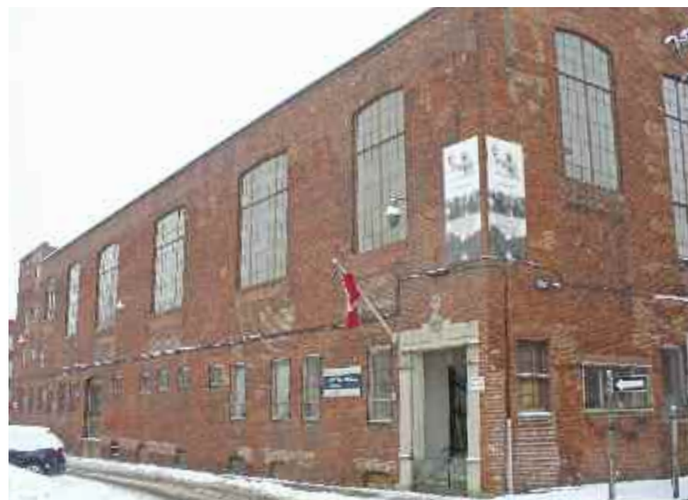
The Hillside armoury, March 28.
