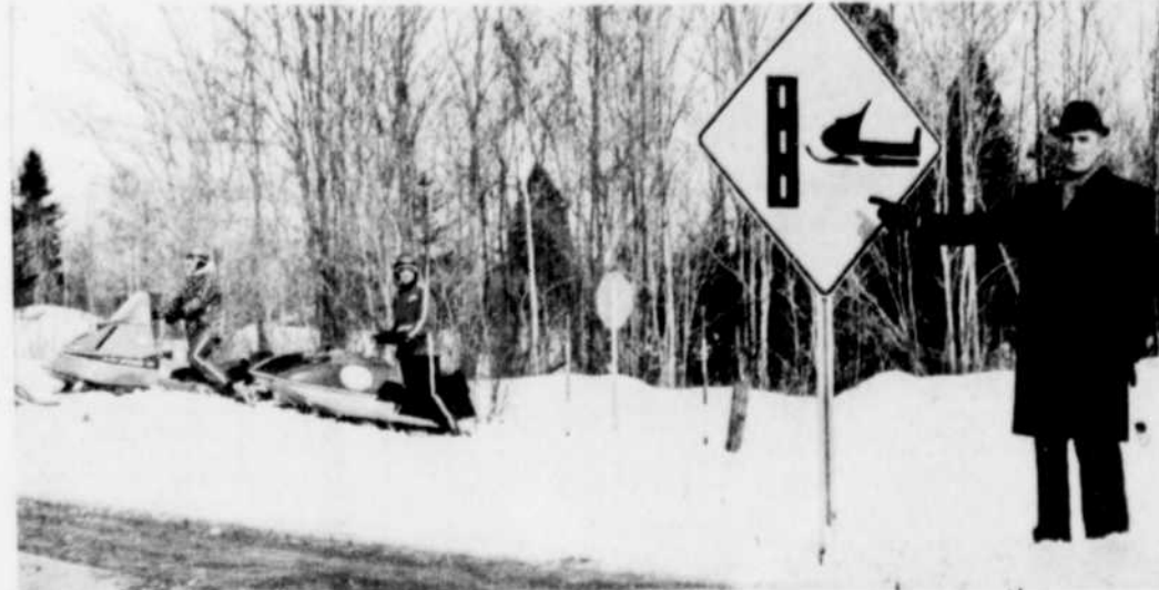
NEW — Roads and Public Works department minister Bernard Pinard indicates a new directional sign that the government installed
