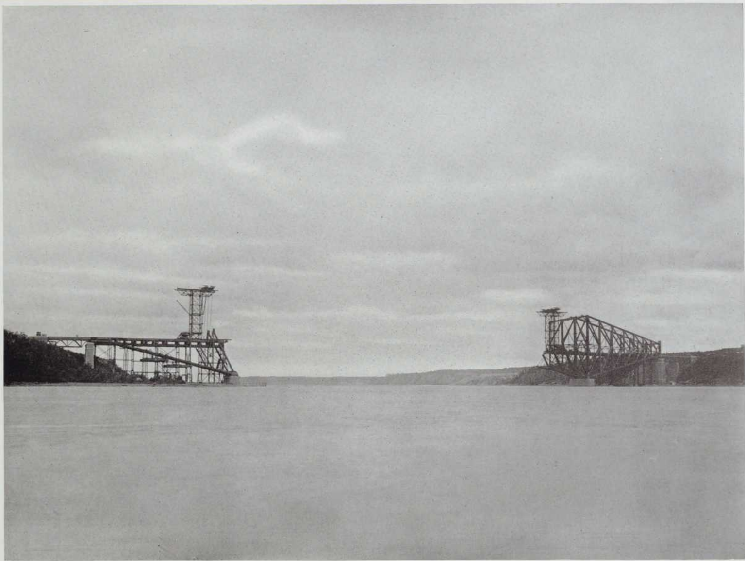
42—Progress of erection, August 18, 1915
