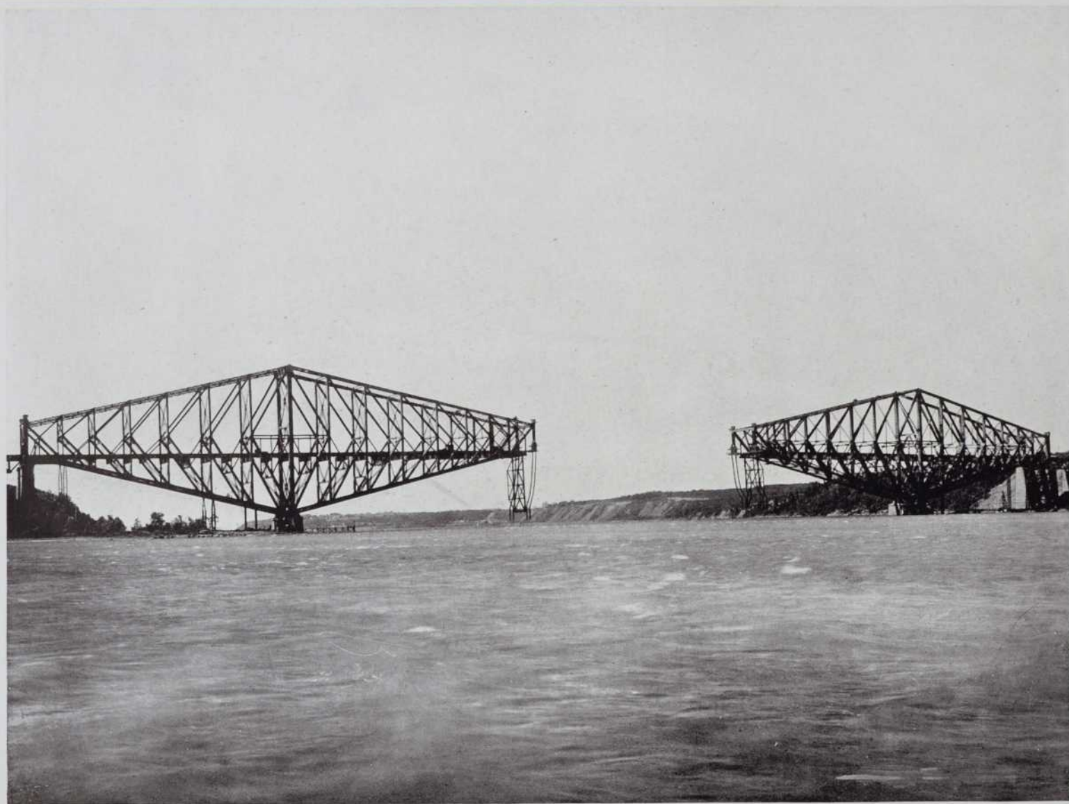
47—Progress of erection, August 11, 1916
