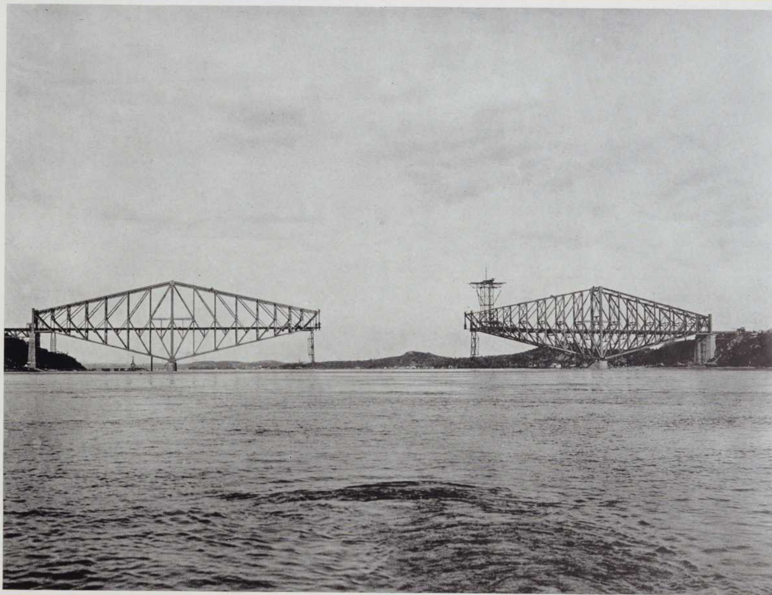
46—Cantilevers completed, hoisting apparatus partly assembled
