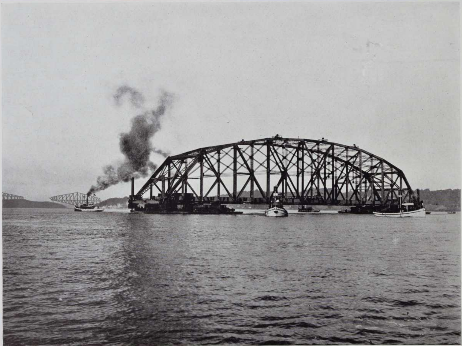
57—The suspended span being guided up the river
