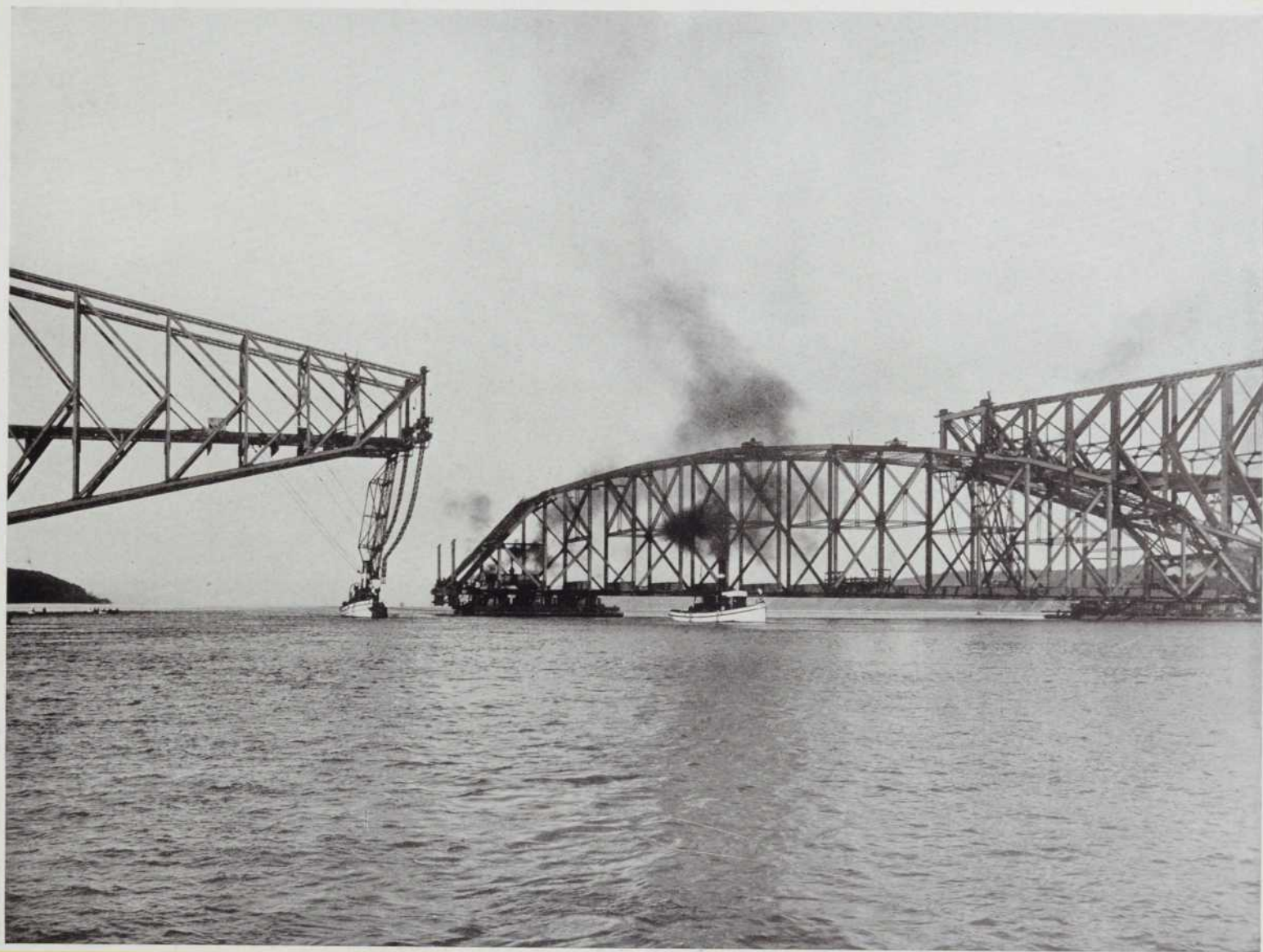
58—The suspended span being guided to position
