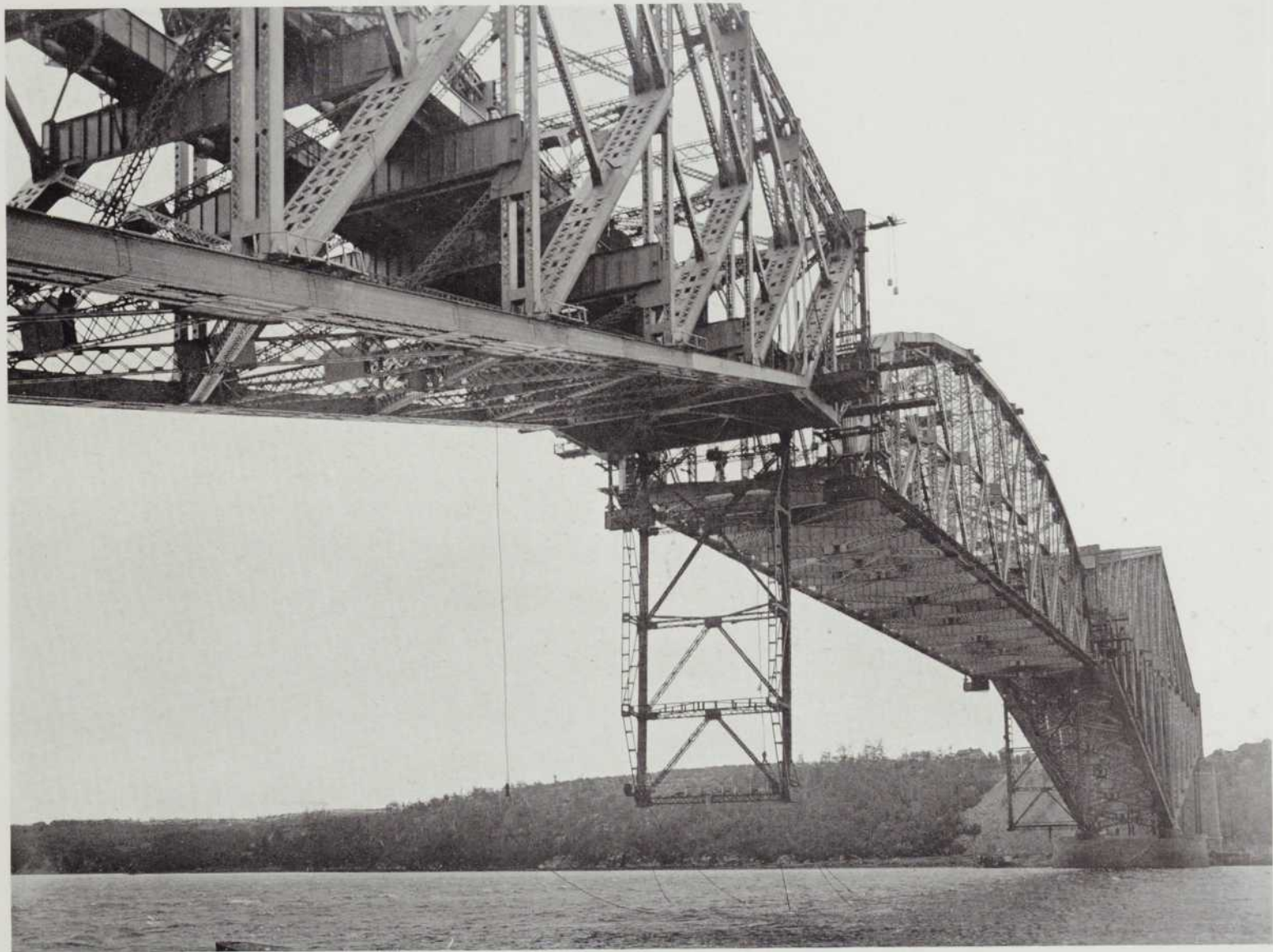
68—The suspended span higher up, September 19th, 1917
