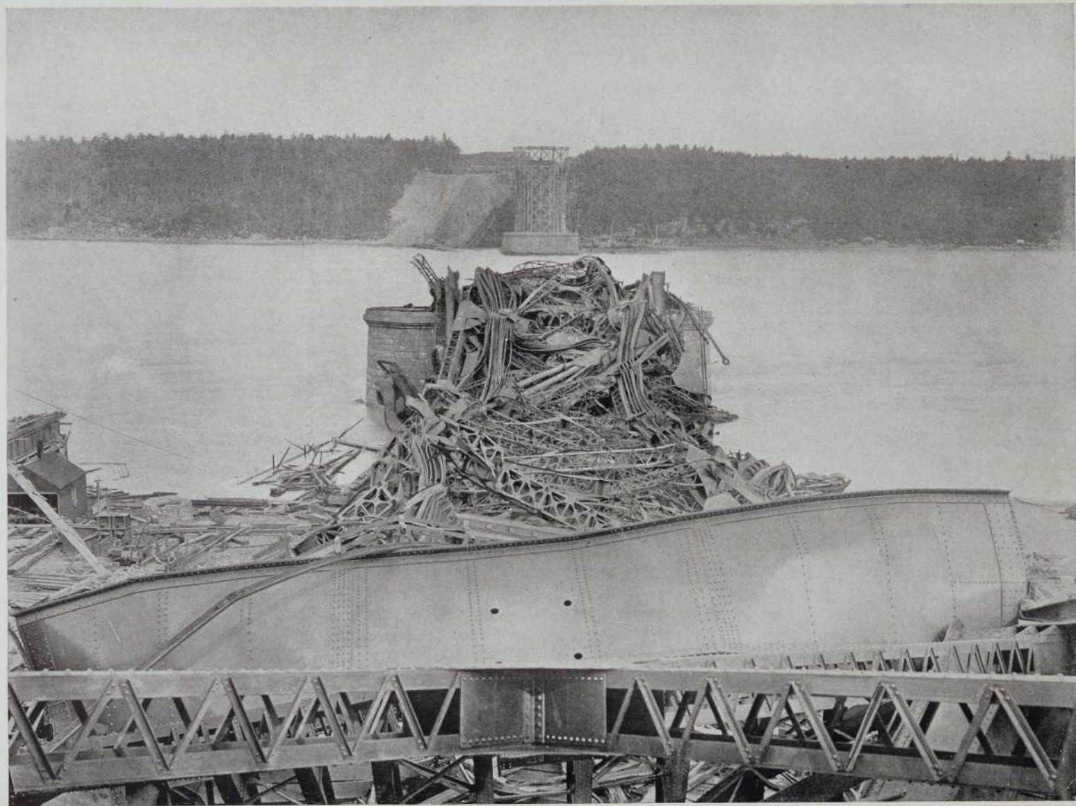
7—General view after the collapse from the anchor pier Northwards
