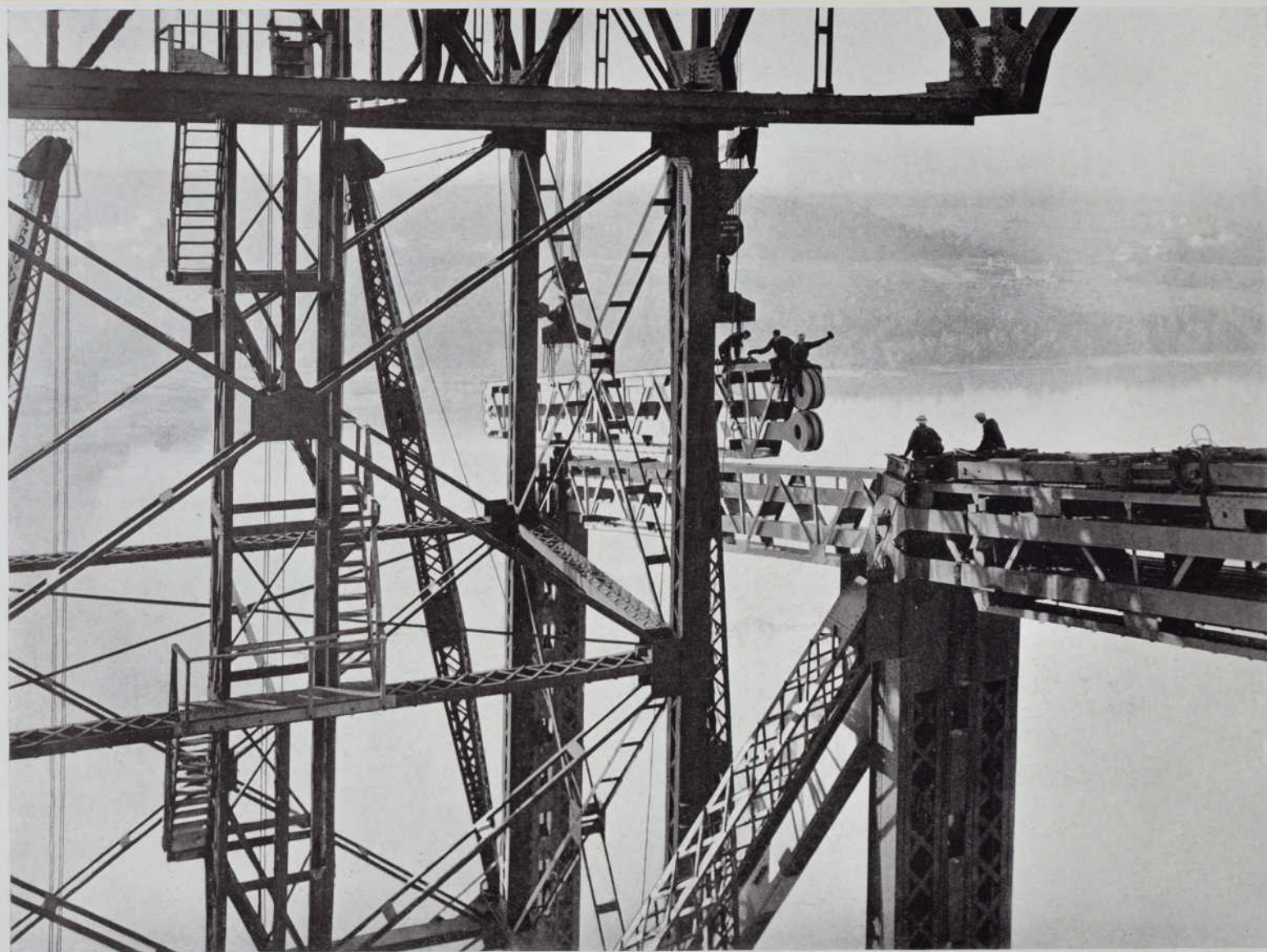
39—Placing the upper chord eyebars of the cantilever arm
