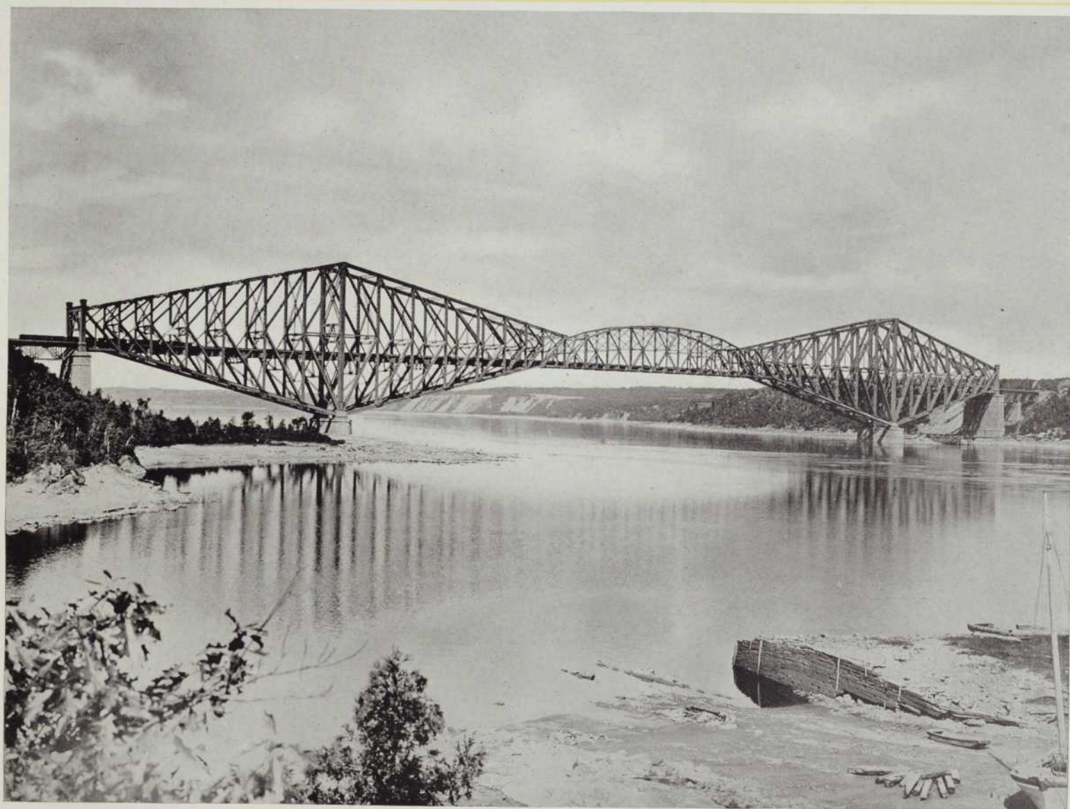
80—Completed Bridge from Chaudiere Wharf
