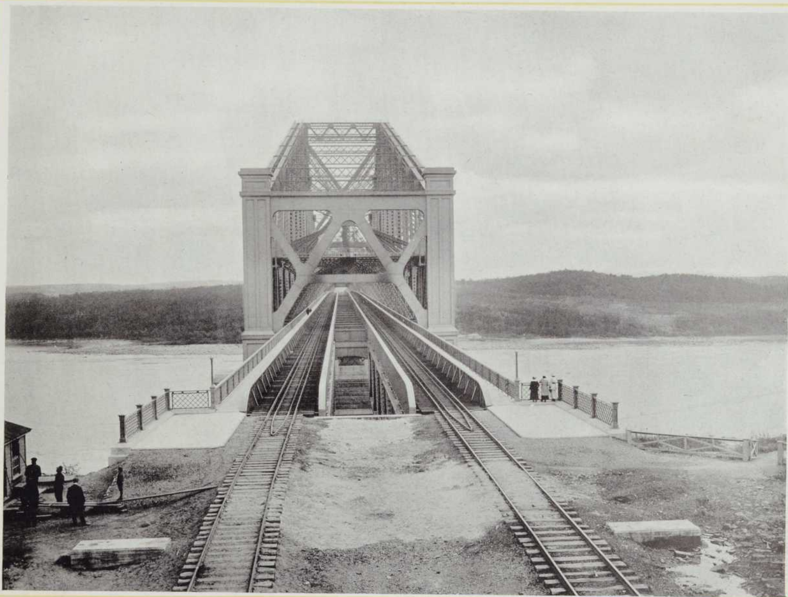
78—End view of the Bridge
