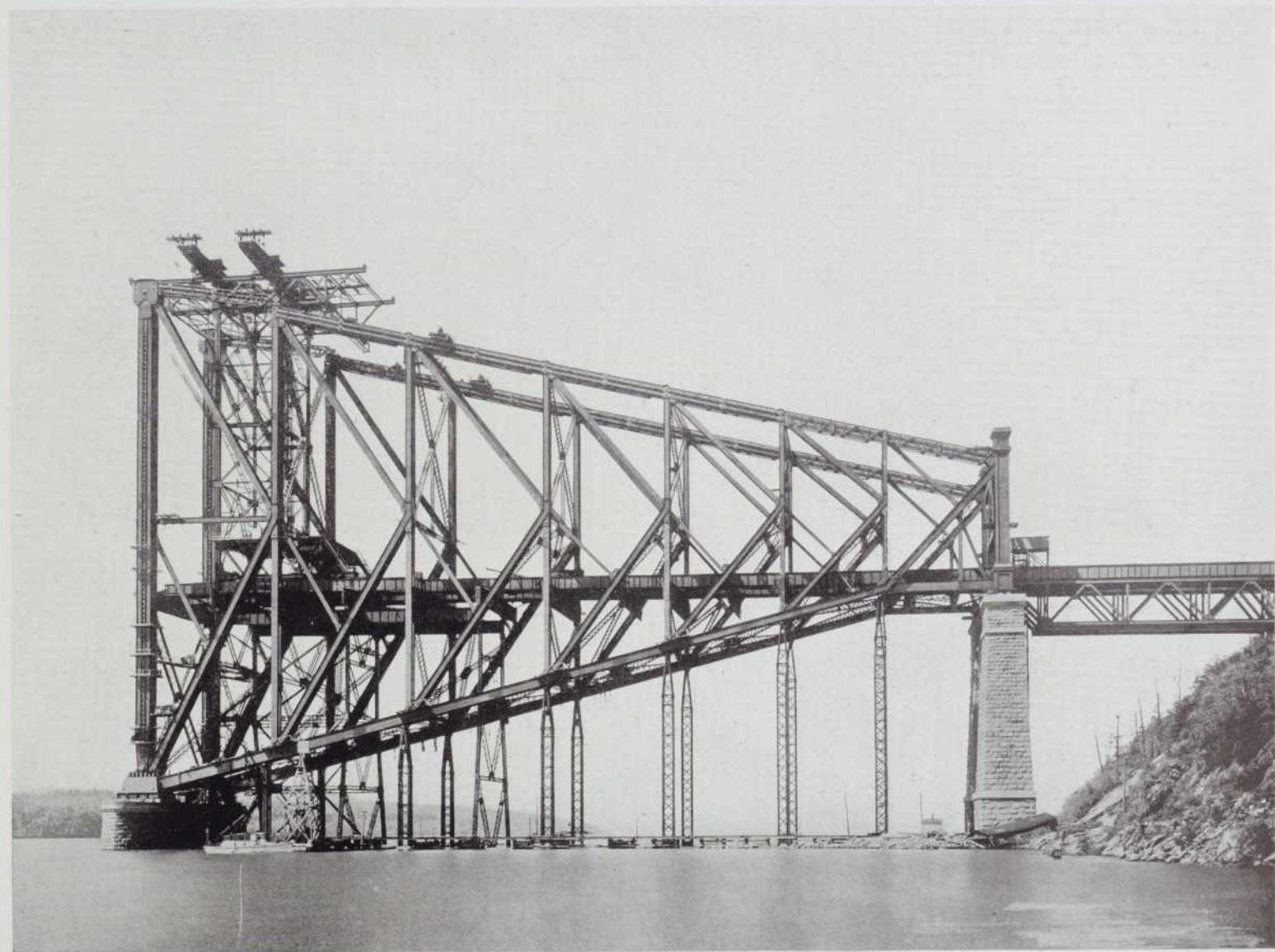
30—The erection of the North Shore anchor arm completed June 7th, 1915
