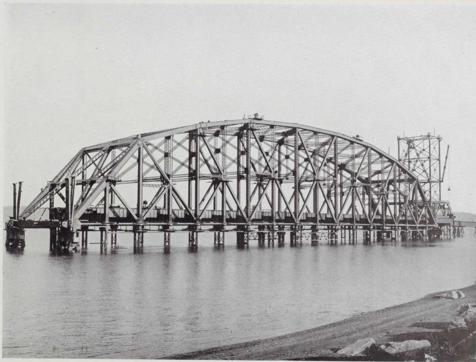
48—The suspended span erected on falsework at Sillery
