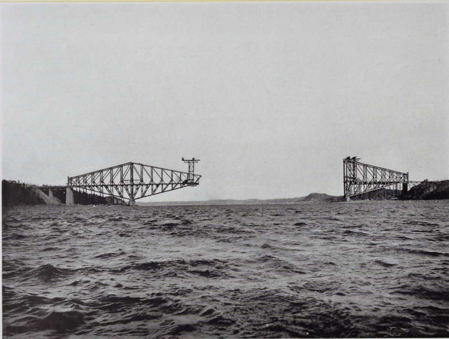
45—Progress of erection at the close of the Season 1915
