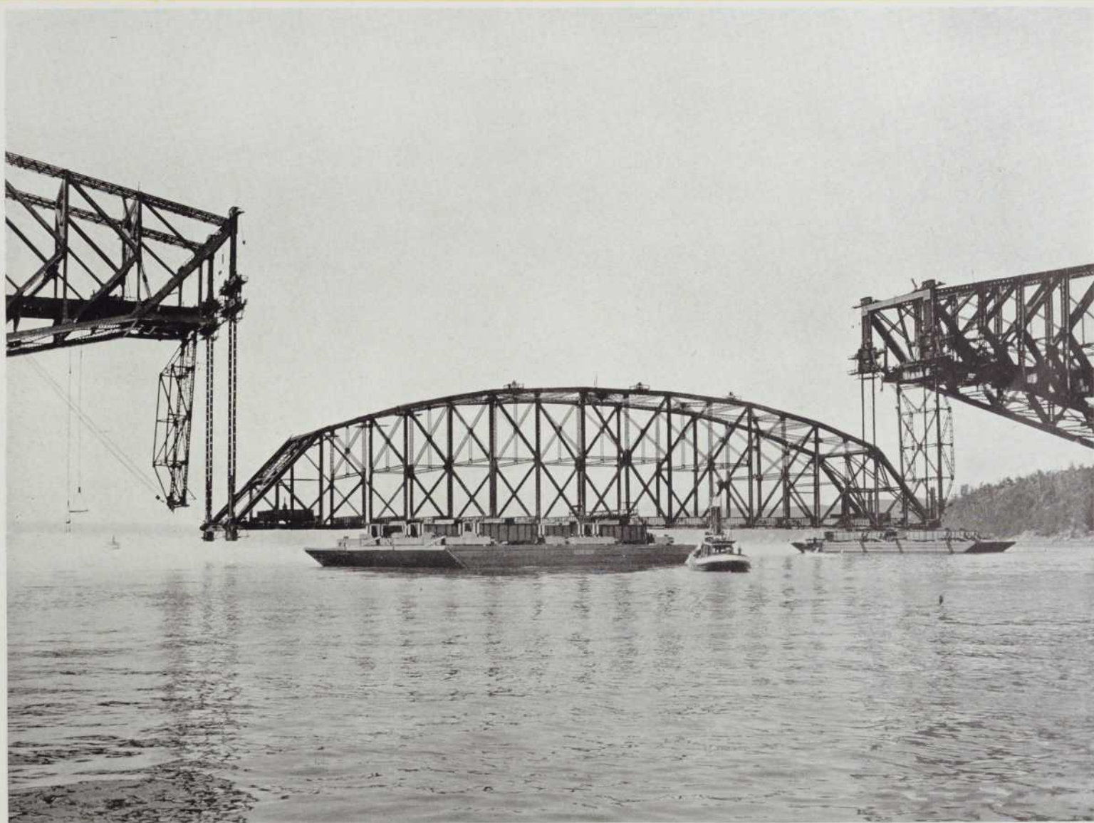
60—The suspended span carried by the hoisting chains; scows floating out
