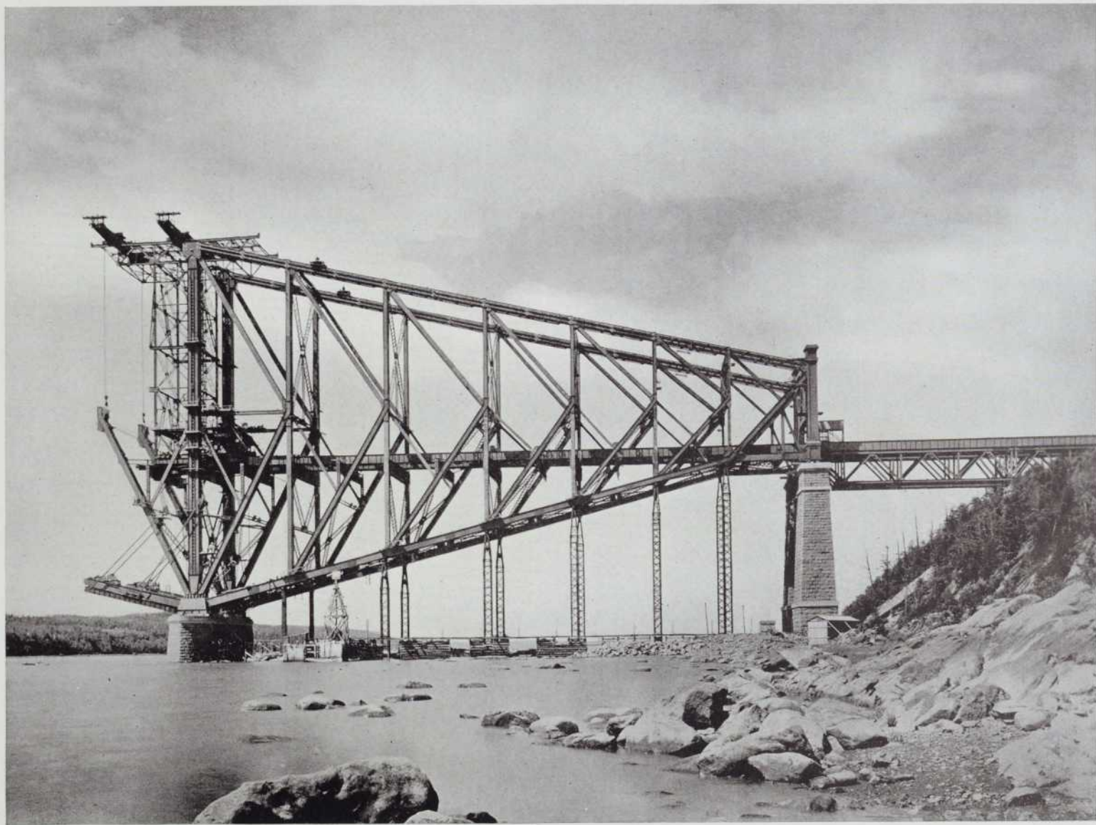
32—Half panel of the cantilever arm erected with the members of the outer half of the panel in place
