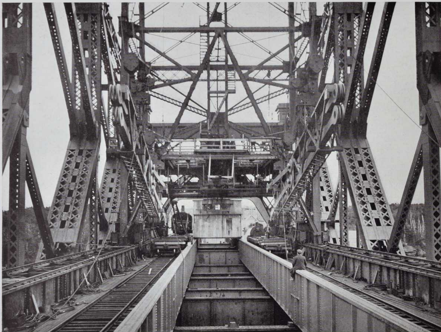
37—Lifting the upper chord eyebars assembled in permanent supporting lattice box girders. Also shows the floor system, the traveller tracks and the switch house
