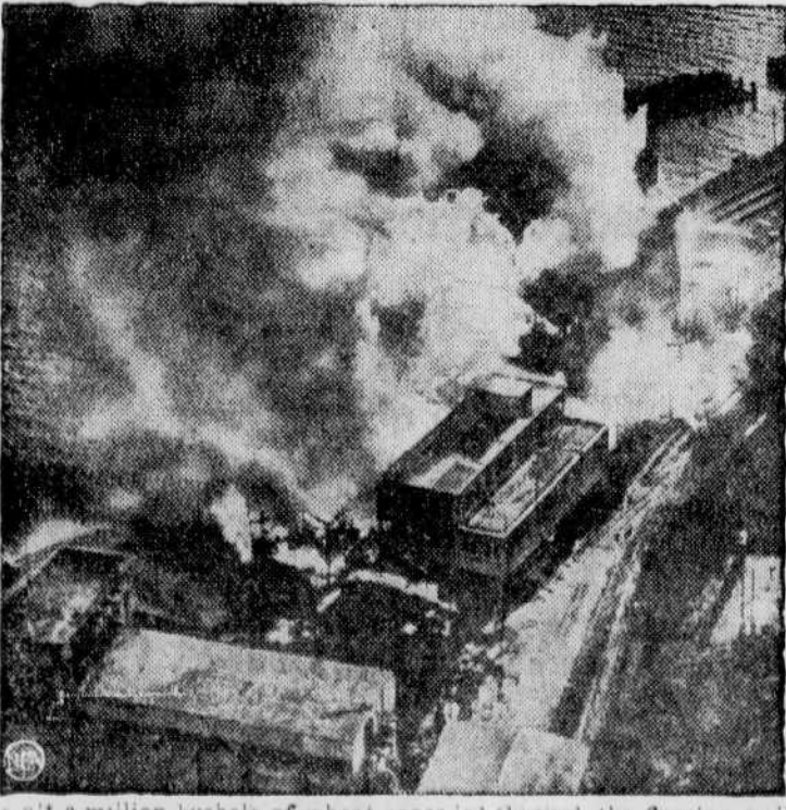
A half a million bushels of wheat cascaded through the flaming walls of three grain elevators (above) during a million dollar fire at the Centennial Flour Mills, Tacoma, Wash. Blaze apparently started from a defective electric motor.
