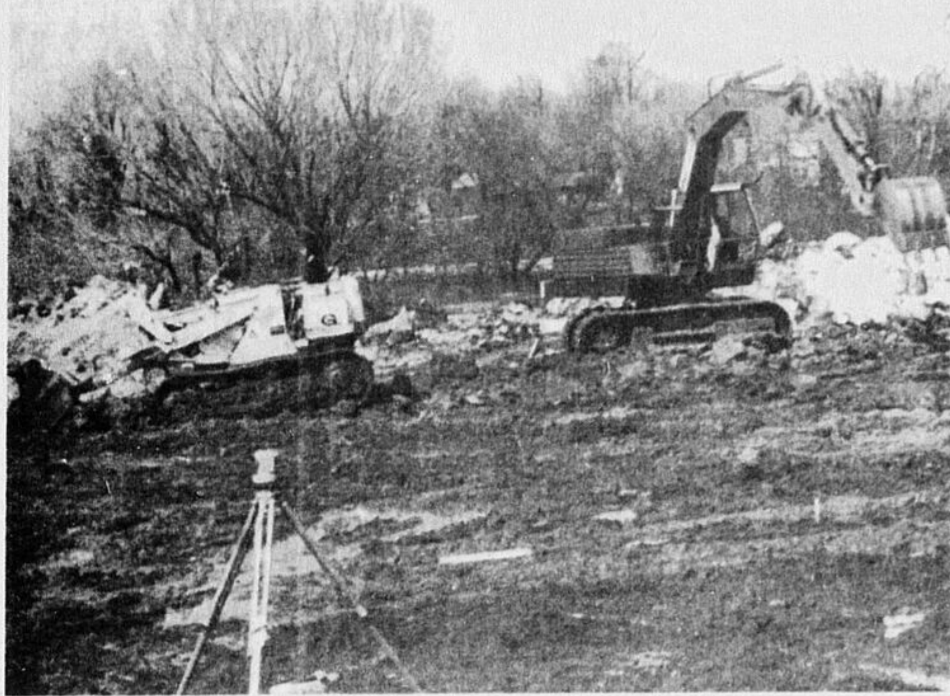
Excavation work began in Ormstown this week on the community's new swimming pool. Complete with chalet and other amenities, the pool will cost about $55,000. Situated on Lot 631 on the north side of Roy St., it is scheduled to begin operations at the end of May.
