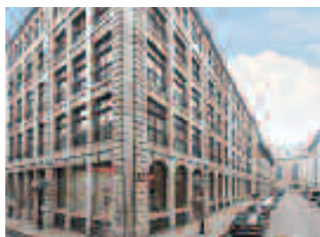
58 DE BRÉSOLES, LOCAL I, OLD MONTREAL $975,000 Unique commercial condo of 3,360 sq ft
