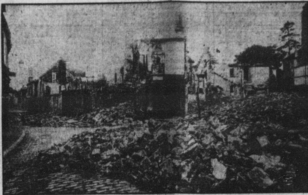
The picture shows the scene of destruction in the ancient town of Senlis, which was twice occupied by the Germans, once in their march on Paris and again during their retreat...
