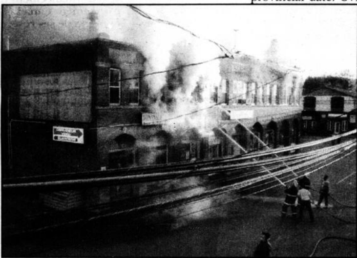
A September 30 blaze destroyed a section of the second storey of Ormstown's historic Walsh Building. (Gleaner file photo)
