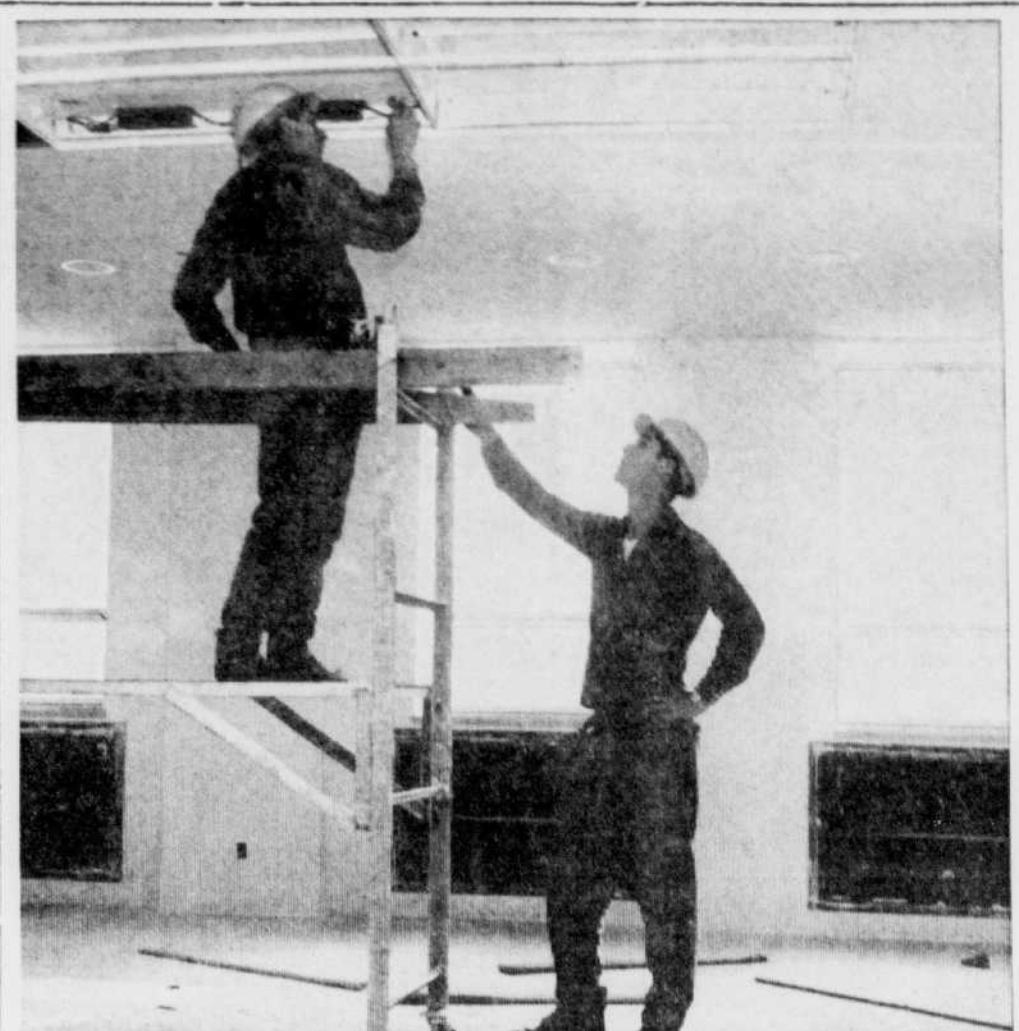
TESTING THE LIGHTS — Gerard Gaudreault, of Sherbrooke, (on scaffold) and Lucien Bourbonnais, of Sherbrooke, are checking the lights in one of the offices in the new U of S medical building now under construction on Stoke Road. The building is expected to be finished by September 1967. (Record photo by Doug Gerrish)
