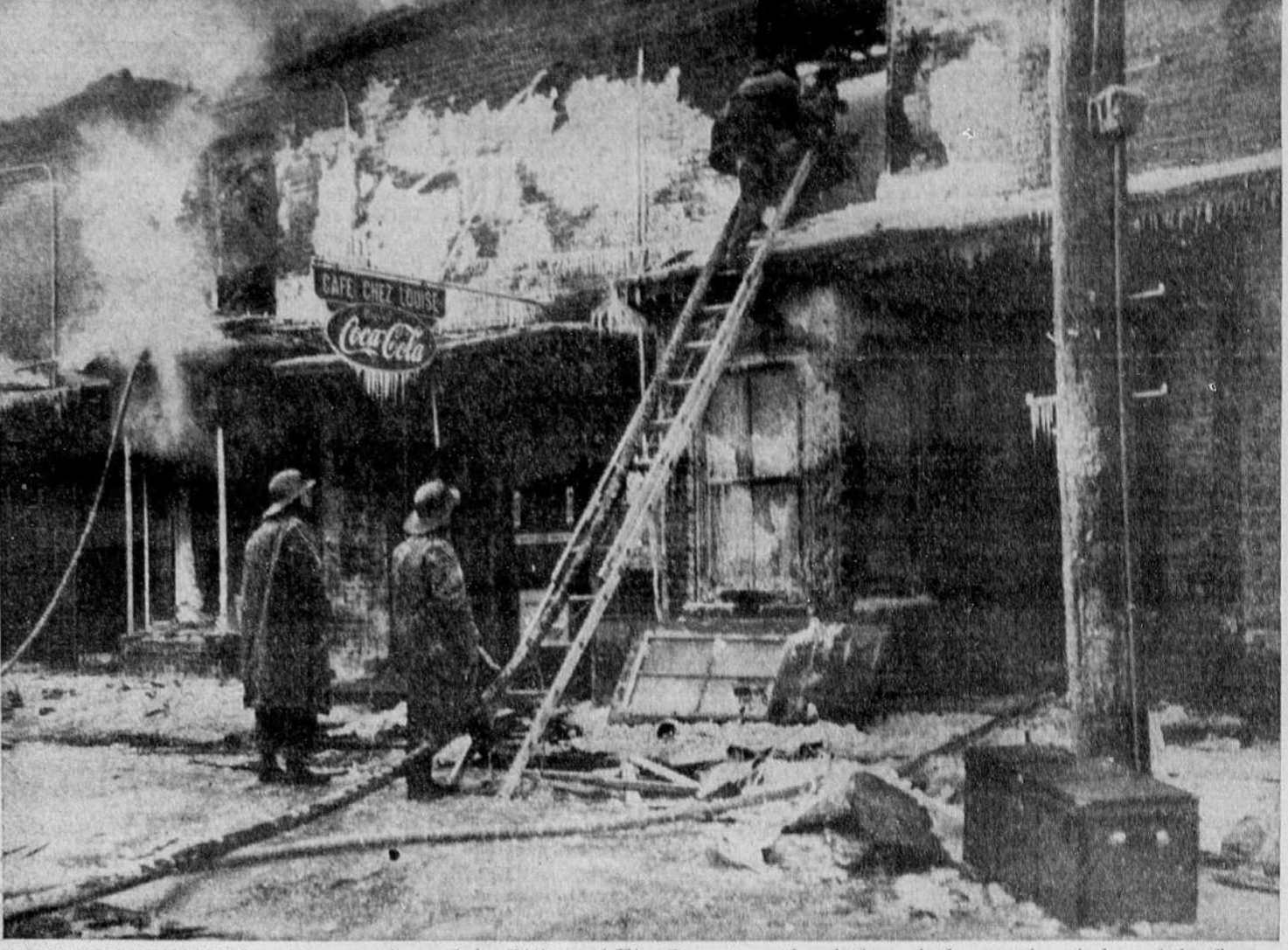
FIREMEN BREAK IN —Two members of the Richmond Fire Department break through the upstairs window of the five-family Main st. tenement that burned stubbornly for four hours Saturday morning. Fire was still raging inside the old building as this picture was taken. Richmond brigade won high praise for their prompt arrival and determined bid to stem blaze which caused damage estimated at $50,000. (Record Photo by Pierre Rochette)
