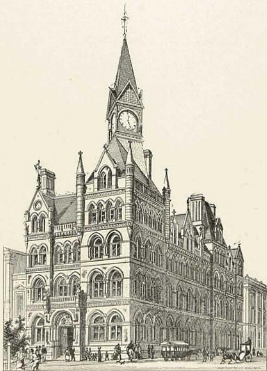
CANADA LIFE ASSURANCE COMPANY'S BUILDING, HAMILTON.
