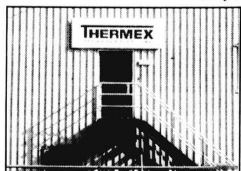
The deserted Thermex plant in Beauharnois.
