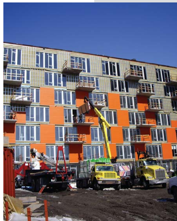
Building the M9 project, in sight of the Bonaventure Expressway
