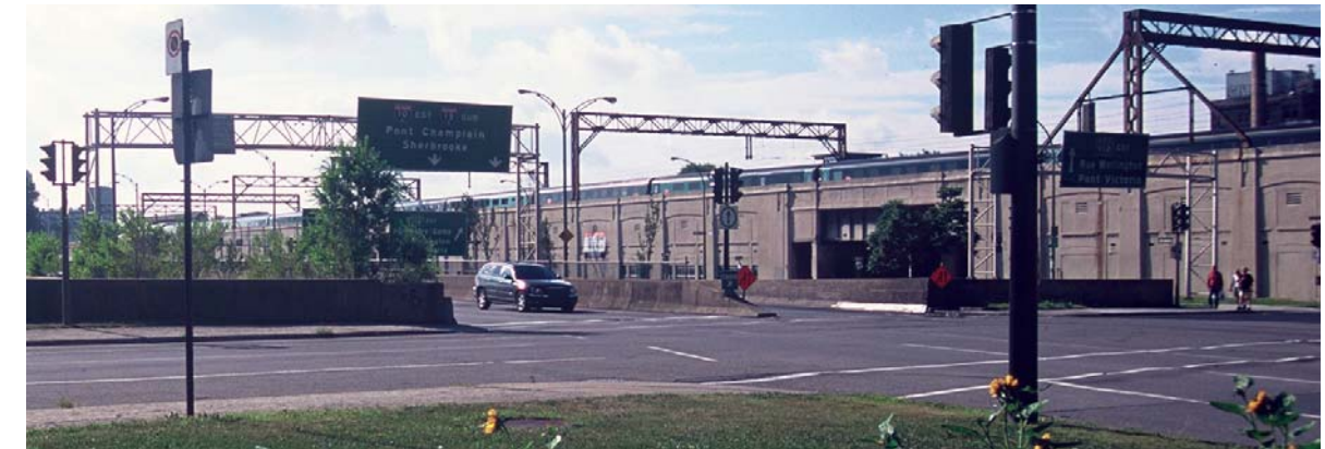
Current view of rail viaduct at Notre-Dame St
