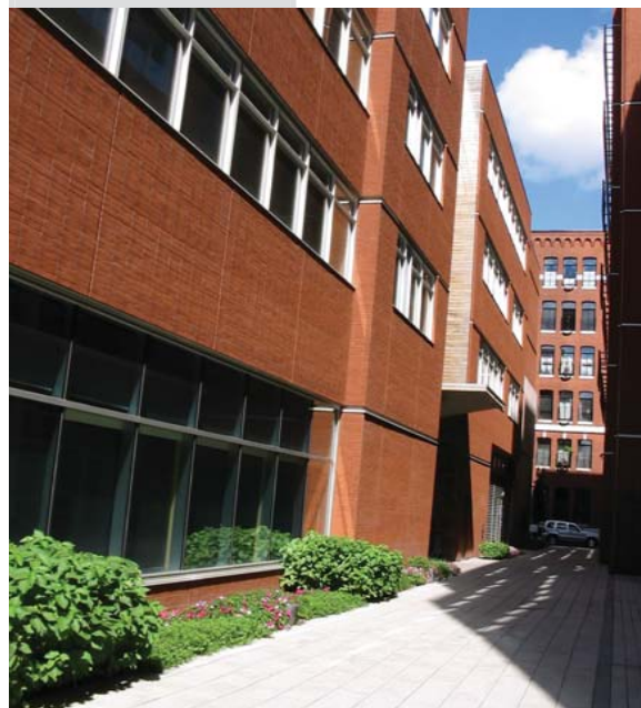
Pedestrian walkway between King and Queen streets, Cité Multimédia
