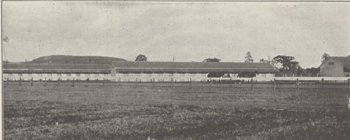
AT A MEET OF THE MONTREAL JOCKEY CLUB—The stables on the Race Course at Blue Bonnets. They are so constructed as to allow the jockeys, stable boys and attendants to have a full view of races going on.
