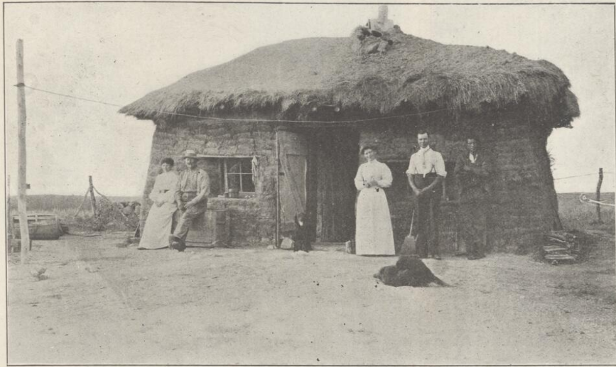
A Settler's Home on the Prairies in Western Canada. It is constructed of blocks of turf, and thatched with straw, and it is far more comfortable and inviting than it looks.
