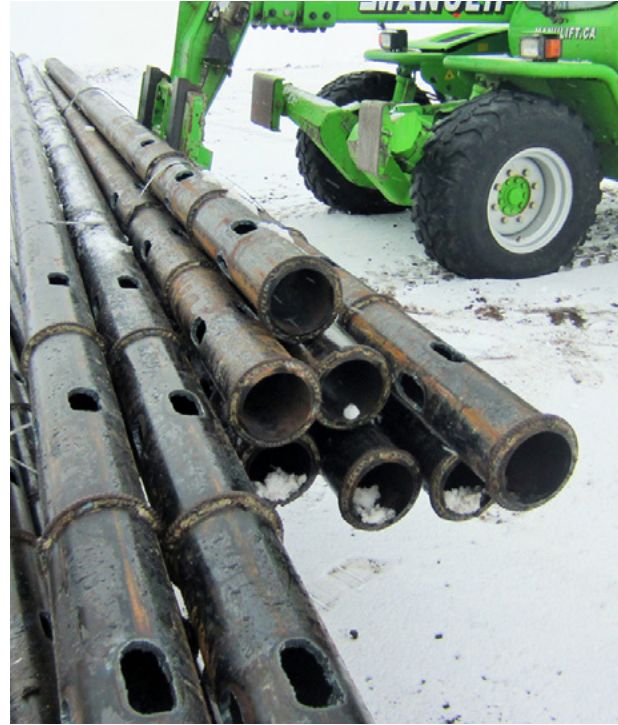
Figure 10: Delivery of piles to the construction site
