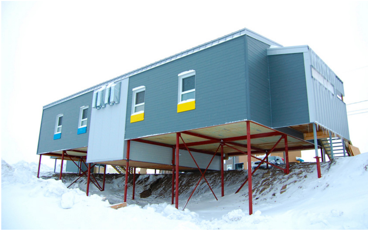
Figure 8: North face of the prototype
