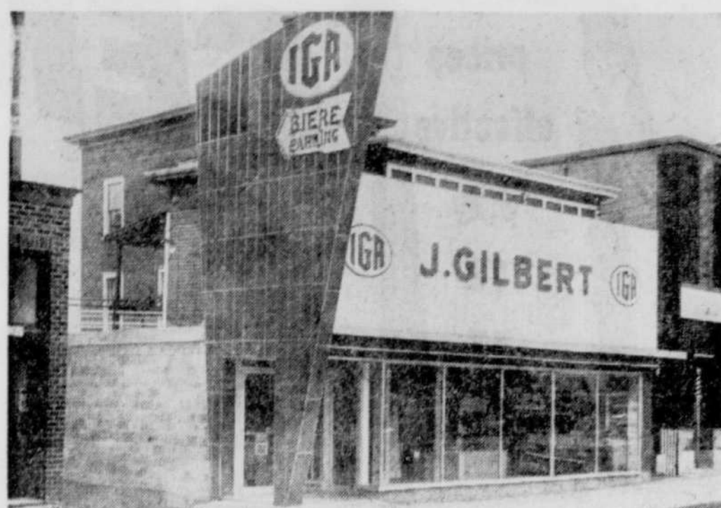
GILBERT IGA RENOVATED — Pictured above is the facade of the Gilbert IGA store, re-opened last week following extensive renovations. Location of the store is on Alexander street.
