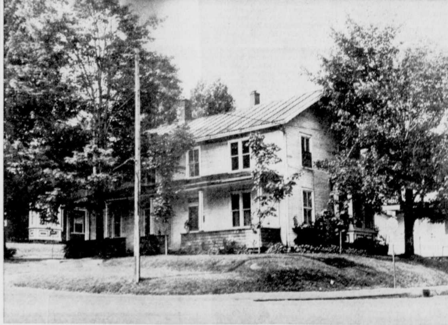
LANDMARK DOOMED — One of the oldest residential properties in the West Ward, this two-family house at the corner of Short and Belvedere streets will soon be demolished to make way for a gasoline service station. (Record Photo by Gerry Lemay)
