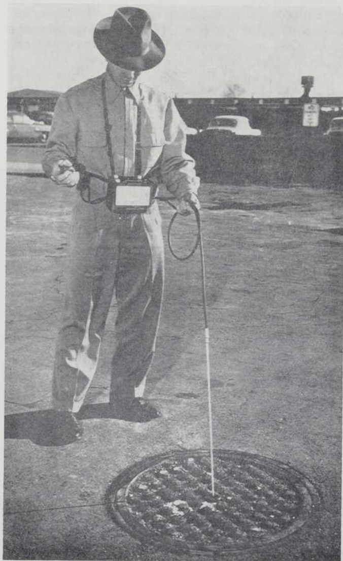
NEWLY DEVELOPED COMBUSTIBLE GAS INDICATOR IS USED TO CHECK ATMOSPHERE IN A MAN-HOLE.
