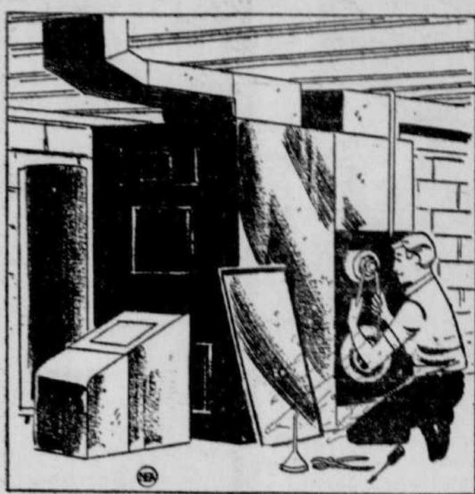
Checking belt tension of the furnace's motor-fan unit is but one of many maintenance tasks that takes minutes, saves dollars.
