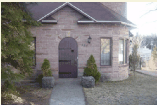
Red standstone of the Robitaille Formation used to manufacture dimension stone in Saint-Mathieu
