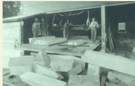
Workshop onsite at the Missisquoi Marble quarry in the 1930s Source : advertisement for the Missisquoi Marble and Stone Corp.
