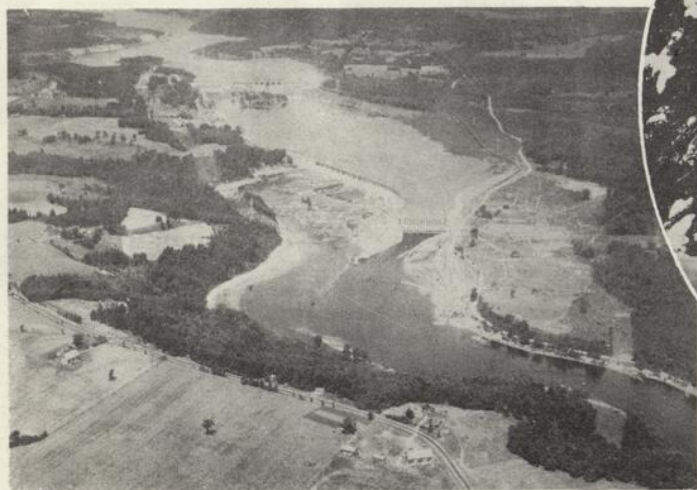
Power development on the Gatineau River as seen from the air. These dams at Farmers and Chelsea Rapids will develop 300,000 h.p. of energy
