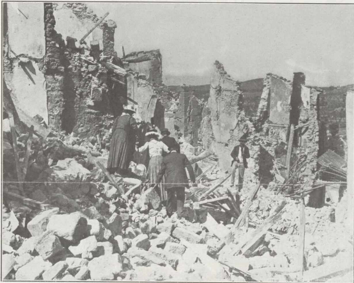
THE HAVOC WROUGHT BY THE RECENT EARTHQUAKE DISASTER IN FRANCE—Sightseers among the ruins of one of the largest houses in Rognes.
