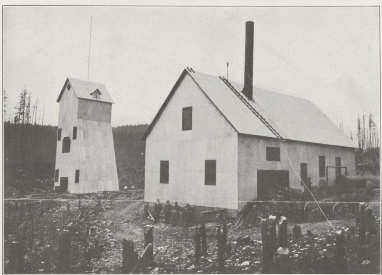
PROGRESS IN THE SILVER COUNTRY—The up-to-date buildings erected by the Otisse-Curie power plant at Montreal River.
