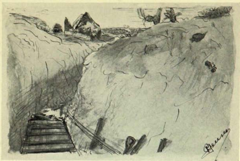
VIA GELLIA COMMUNICATION TRENCH.
