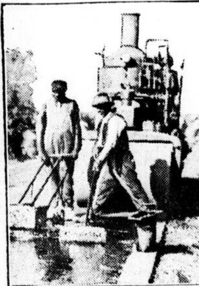
Building a Federal Highway in Virginia.
