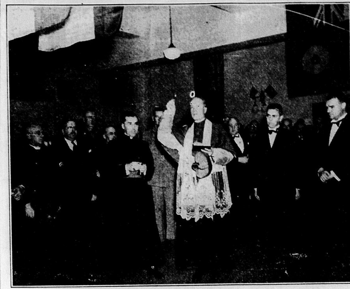
Dedicated to the service of members of His Majesty's Canadian Active Service Forces stationed in or near Montreal, the second local unit of the Knights of Columbus Canadian Army Huts was formally opened this week. It is the twenty-seventh such establishment to be opened in Canada, in addition to units in England and Iceland. His Excellency the Most Rev. Joseph Charbonneau, Archbishop of Montreal, is here shown in the act of formally blessing and dedicating the Hut. On his left is Rev. Canon Lawrence Whelan, chancellor of the archdiocese. On his right is Dr. J. K. Carver, district deputy, Knights of Columbus, and chairman of the Montreal Army Huts Committee; and Emmet J. McManamy, Grand Knight of Montreal Council No. 284, Knights of Columbus.
