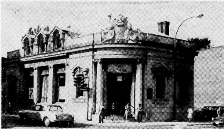
Since early last winter, before the local main postal station was moved to St. Catherine and Olivier from its 56-year-old home, there were indications that "Canada Oldest Bank" had some new and modern ideas for its valuable and strategic location in a thriving and renewing Westmount business section and diagonally opposite prestigious Westmount Square. Its traditional-style premises (above) furthermore, were becoming cramped.
