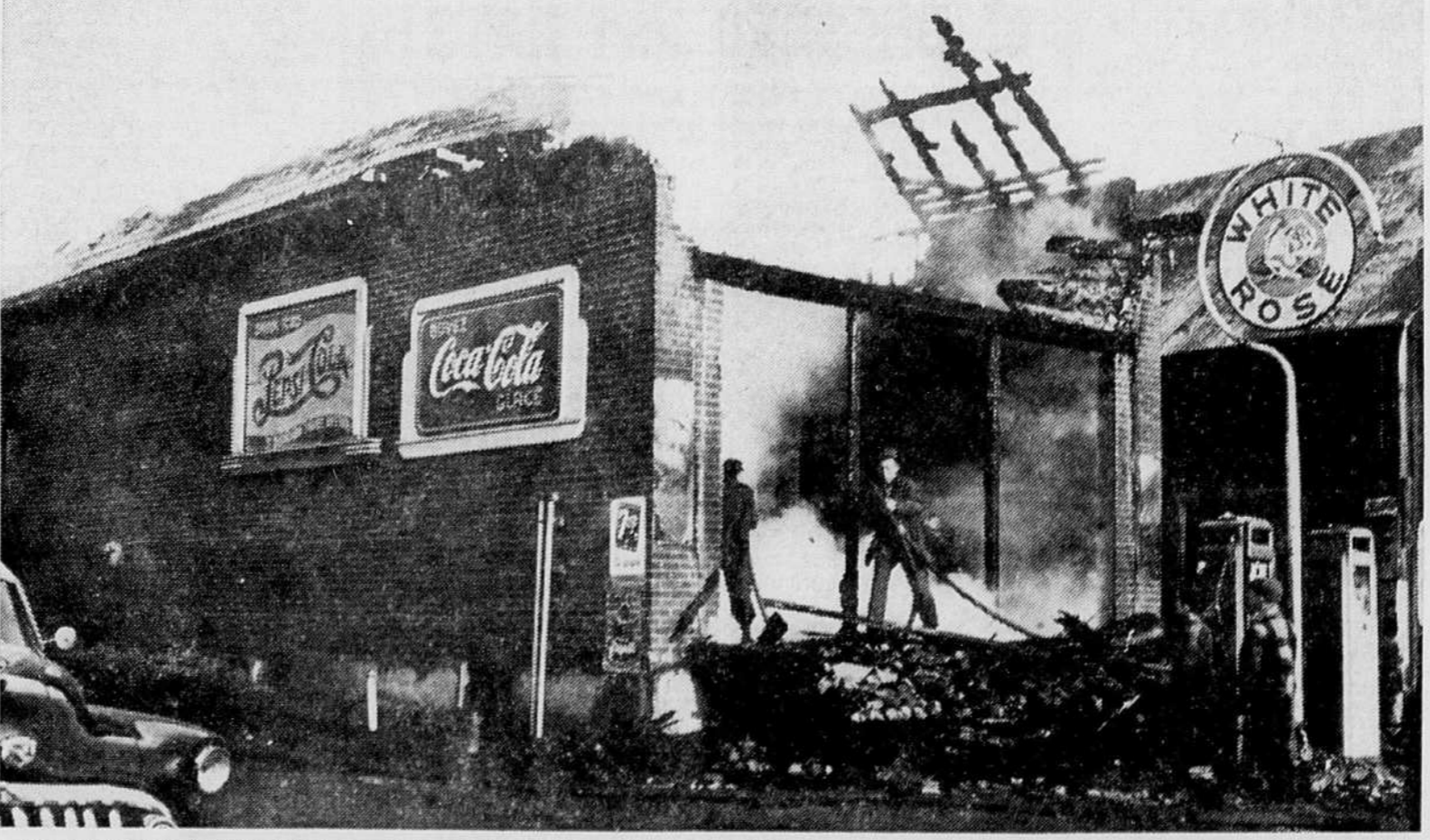
ASCOT CORNER FIRE: All that remains of the Rodrigue Bergeron general store and gasoline station, burned out in a fire early this morning, is shown above. Damages estimated at $35,000 were caused in the fire whose origin is not determined. (Record photo by Gerry Lemay).
