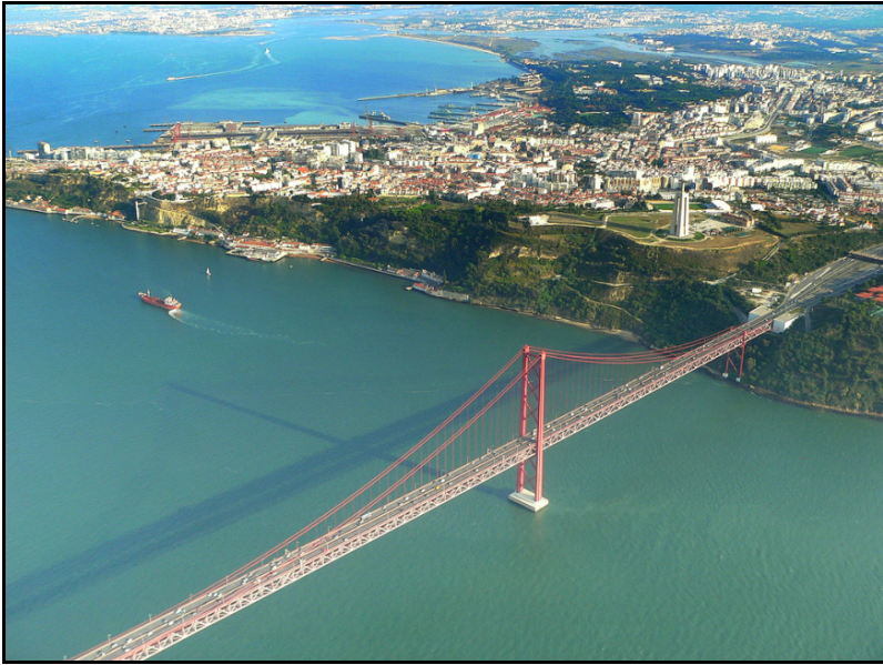
Figure 3.29: April 25 Bridge [referring to April 25, 1974 when the dictatorship was reversed] connecting the city of Lisbon to the municipality of Almada on the left (south) bank of the Tejo River.
