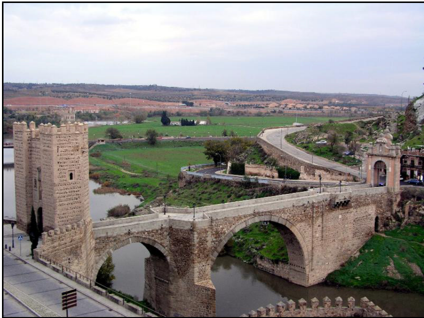
Figure 2.29: Bridge across Tajo River.
