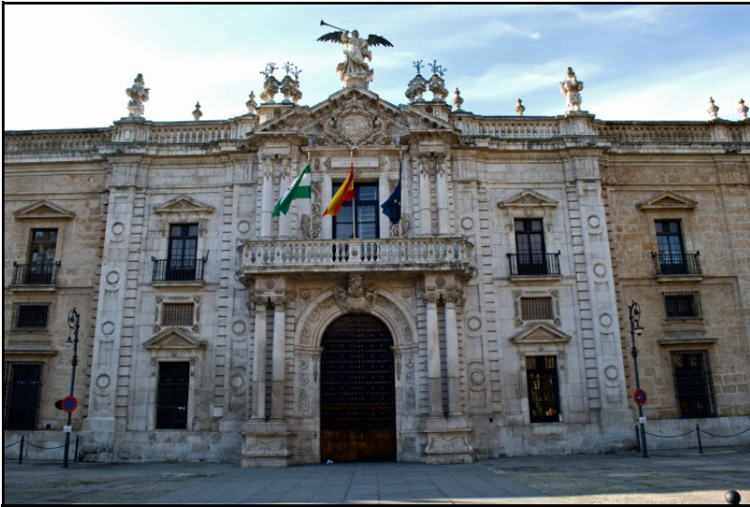
Figure 2.55: Façade of the University building.
