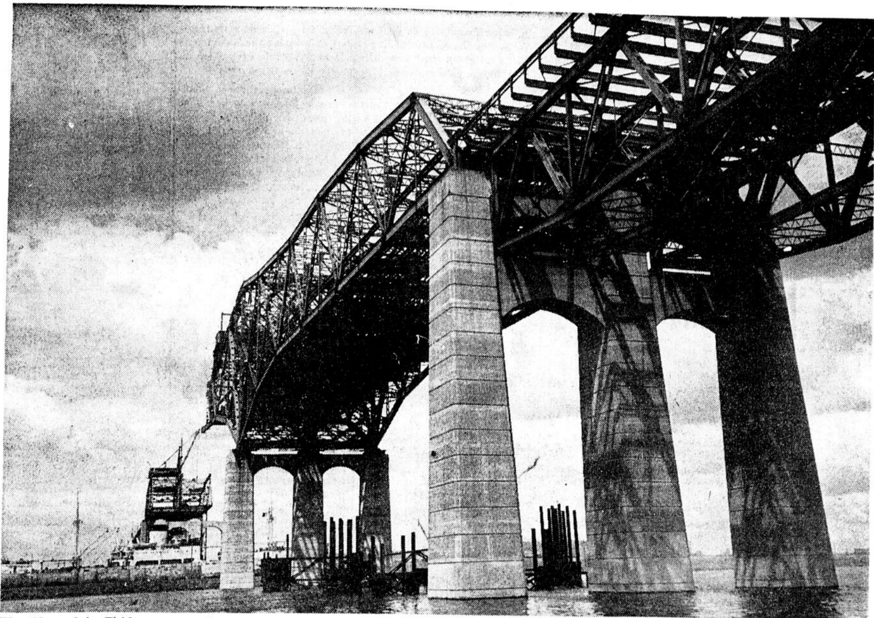
The Champlain Bridge, now under construction between the South Shore and Verdun, via Nun's Island, presents a rather spectacular sight from the vantage point of a boat in the St. Lawrence Seaway channel from where this photo has been taken.
