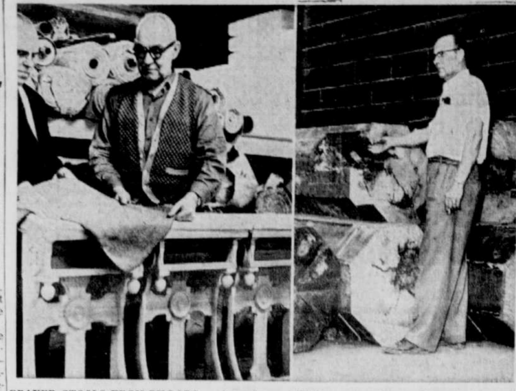
PRAYER STOOLS FROM PILLARS — A workman (right) examines huge yellow pine pillars removed from Montreal's Notre Dame church after they started to rot. The pillars, replaced by concrete columns, were milled into lumber by a furniture firm and converted into the prayer stools shown with Ferand Thibault, (left), president of the firm, and plant foreman Joseph Peterson. Part of the original church built in 1824, the pillars were hewn from trees cut near Cornwall, Ont., and floated down the St. Lawrence River to Montreal.
