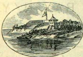
PORT HENRY—MARTELLO TOWER, CEDAR ISLAND.
