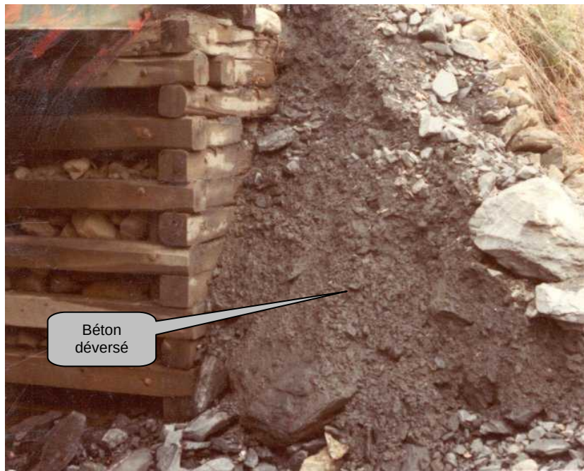
Photo 5.5.3 d) – Protection de talus
