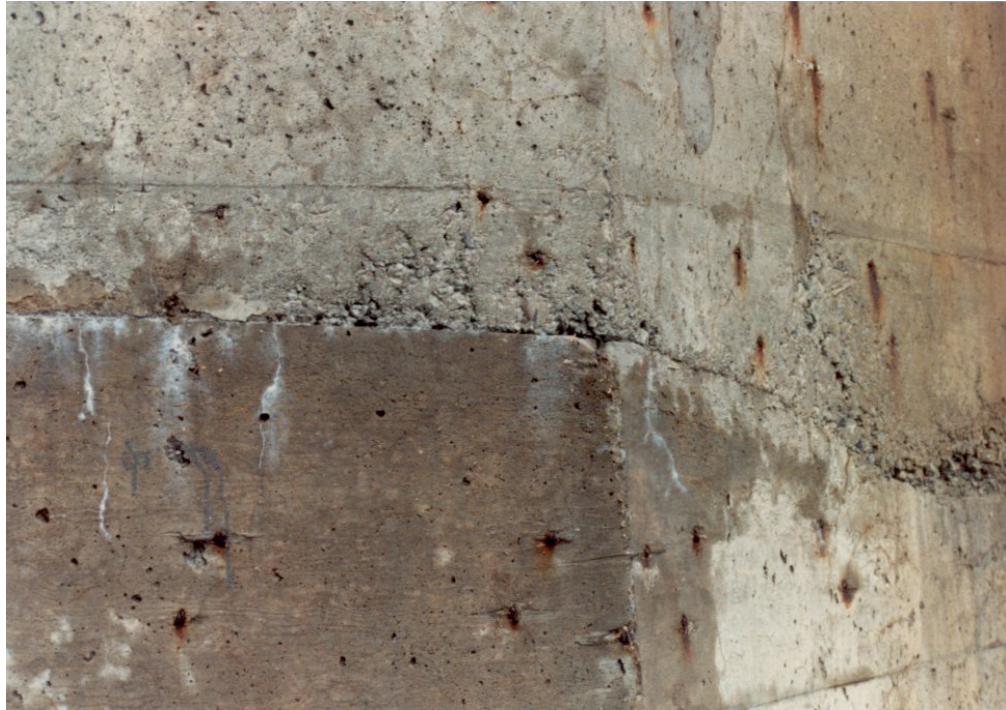
Photo 3.2.8 – Joint froid
