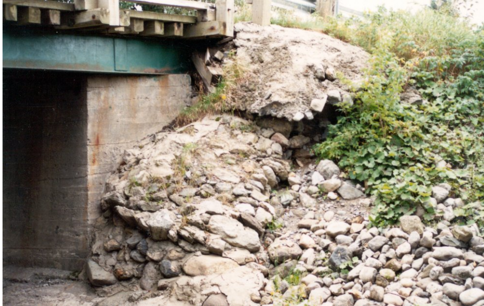
Photo 5.5.3 c) – Protection de talus
