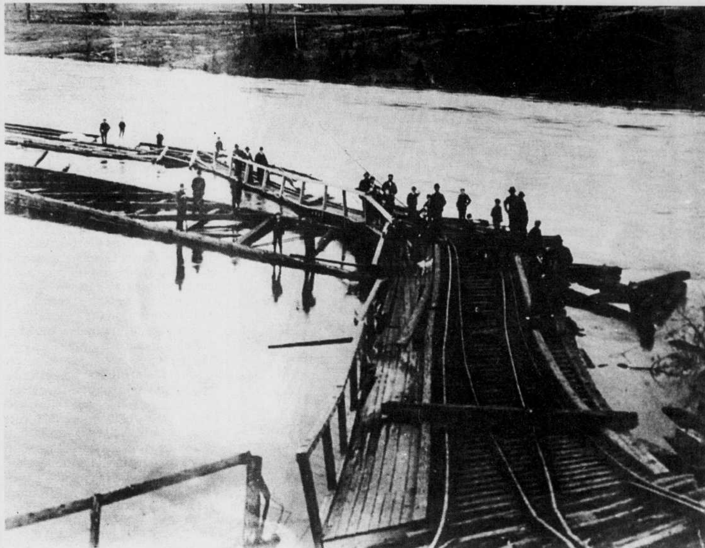
Is this a bridge over troubled water or just a bridge in trouble? Both seem to be fair statements but when and how could this have happened. If you have any information on this photo, please let us know at newsroom@sherbrookerecord.com or by calling 819-569-6345
