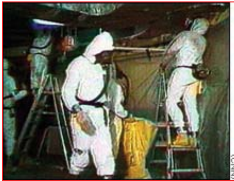
Removal of asbestos
