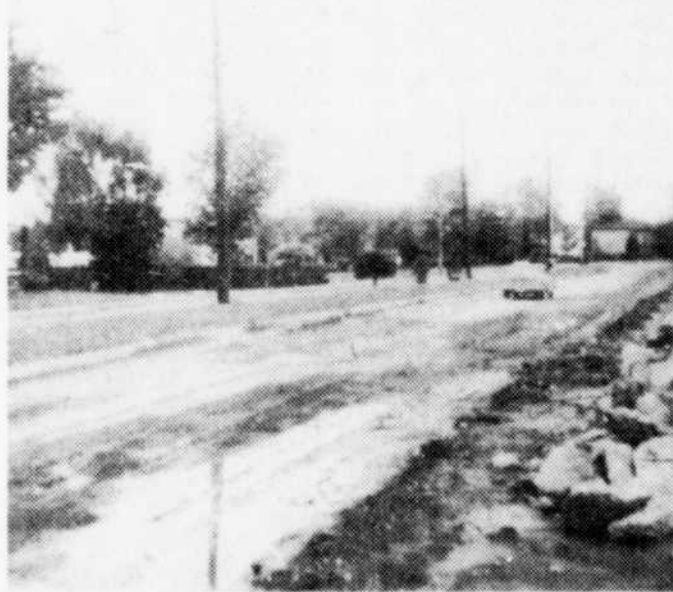
DIEPPE BOULEVARD — Only regular maintenance will be carried out here in Cowansville until work on the street's sewage system is complete.
