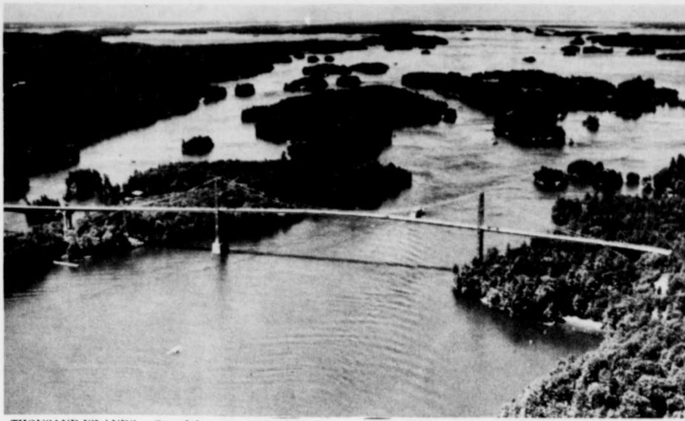
THOUSAND ISLANDS — One of the most scenic sights in North America is the seven-mile, island-hopping five-span 1000 Islands Bridge linking New York State and the Province of Ontario. Seen here is the Canadian suspension
