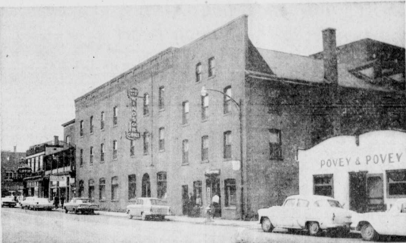
DEMOLITION WORK EXPECTED SOON — The Windsor Hotel, a familiar landmark in downtown Sherbrooke will disappear when demolition crews start work to make way for the construction of a 225-car parking lot. City council recently approved the purchase of the hotel on Depot Street at a cost of $167,000. Also to be torn down are the Surplus Depot, R. W. Mitchell, Povey and Povey establishments.
