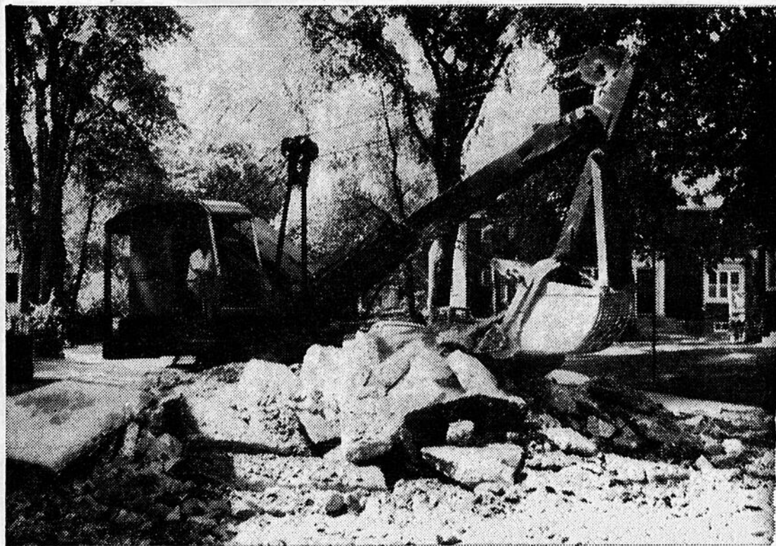
Excavation proceedings started Wednesday on Clarke Ave. above Sherbrooke — the first
