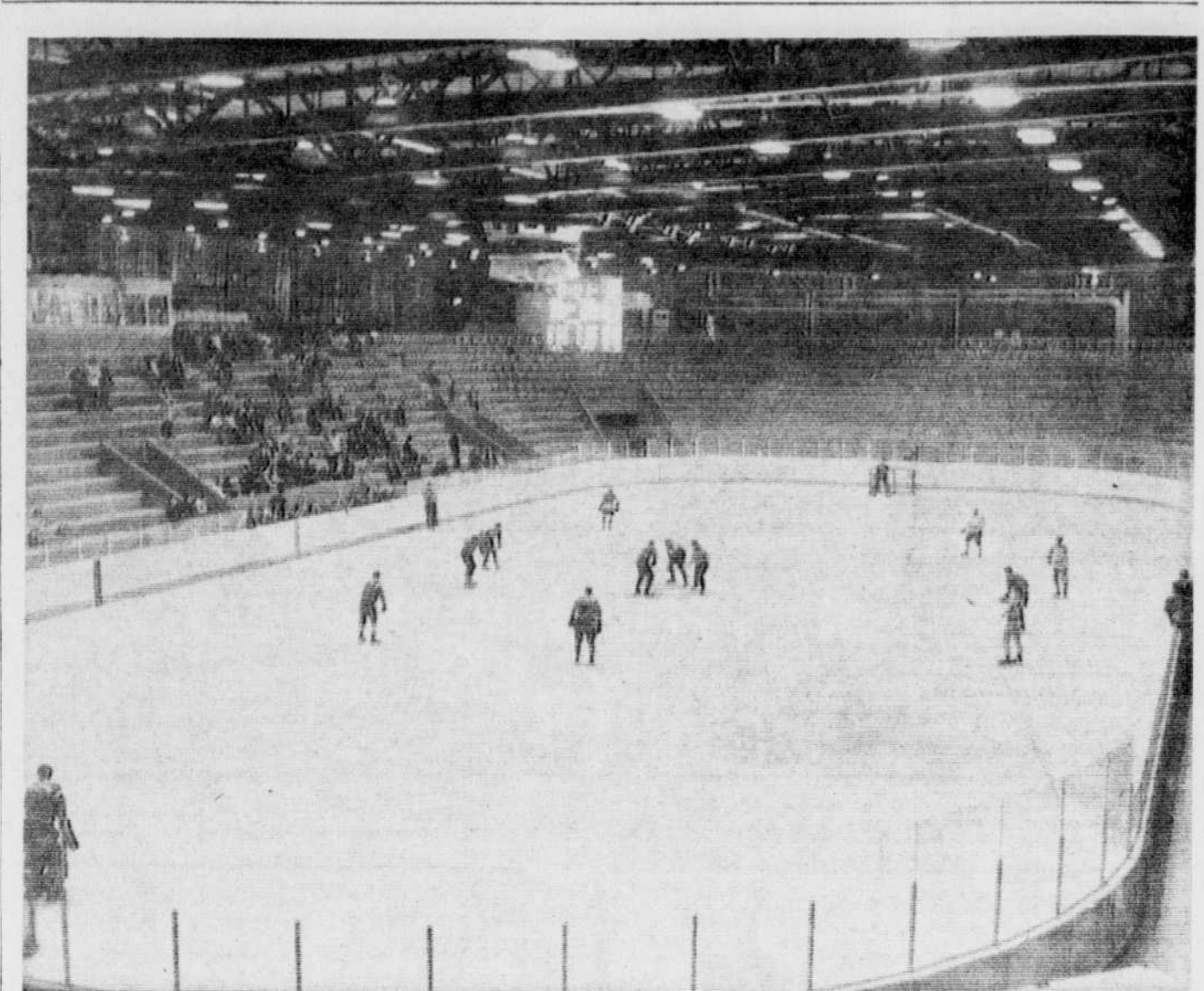
AT LAST — The ice machines of the Sports Centre got their initial test this week when a surface was laid to see if everything was in tip top shape. Shown are above are the men who helped build the Centre enjoying a game of hockey. The Construction squad went down to a 6-4 defeat at the hands of the Architects and Technicians.
