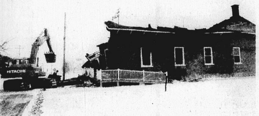
Hinchinbrooke Town Hall after the first last December 13 that destroyed it.
