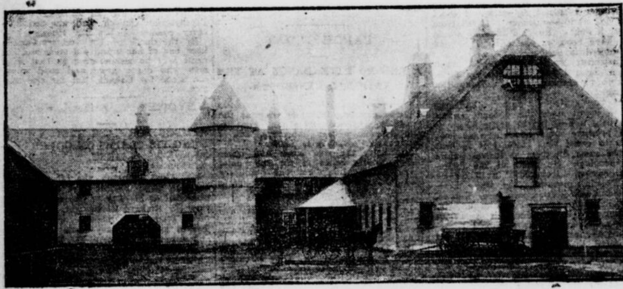
A PORTION OF THE DESTROYED BUILDINGS.
