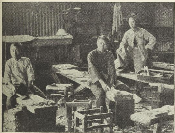
FIG. 5.—Corner of carpenter's shop, New Engineering & Shipbuilding Co. Ltd.,
