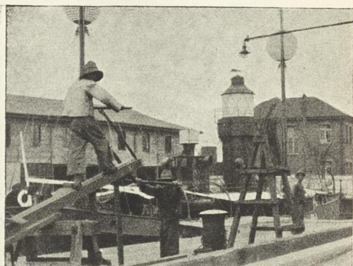
FIG. 6.—Chinese sawing wood for shipbuilding purposes. New Engineering & Shipbuilding Co. Ltd.,
