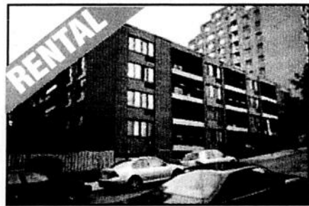
Redpath. In the heart of Downtown. Great top floor 3 bdrm, 2 bath condo, fireplace, garage. $2,500/mo heated.
