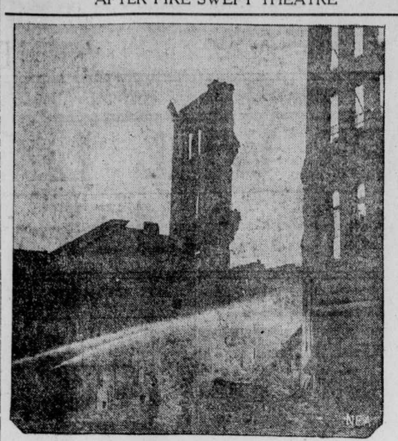
Three people died when fire swept the Gillis Theatre in Kansas City. This picture shows firemen showering water on the blackened walls, which are all that is left of the building. Fortunately few people were in the place at the time.
