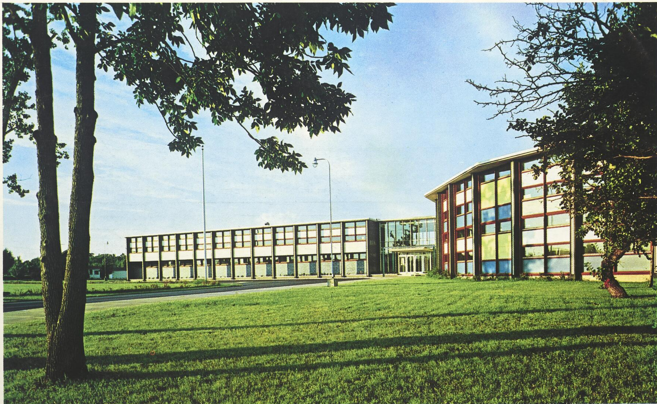
MAIN ENTRANCE, LINDSAY PLACE HIGH SCHOOL
