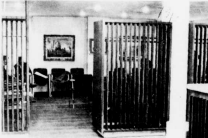
WAITING ROOM OF THE CLINIC
