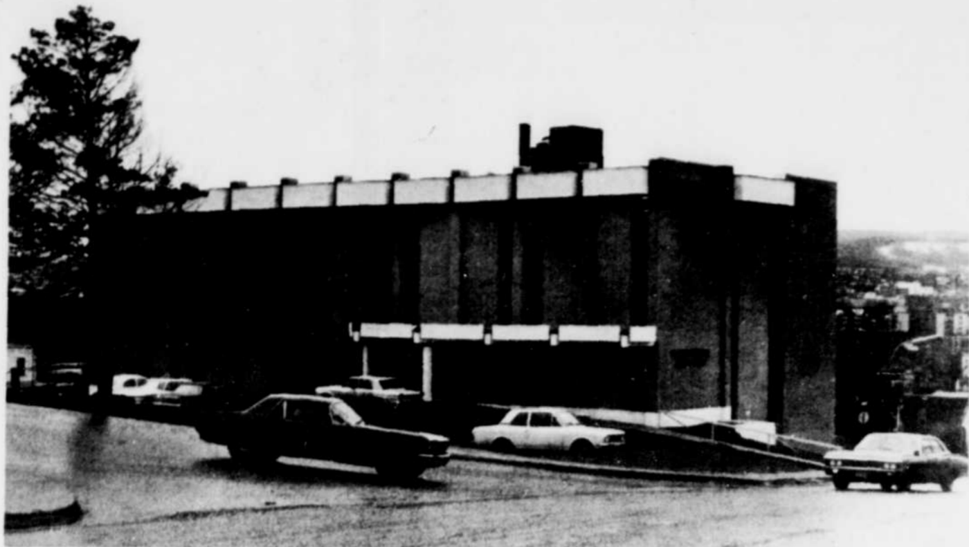
EXTERIOR OF THE NEW ST. VINCENT FAMILY CLINIC
