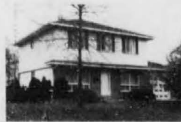
BEACONSFIELD: $89,100 [6] 8 rooms, 4 bedrooms, family room, fireplace, main floor, beautiful deck, nicely decorated. Nicole Gauvreau 754-7540, 697-2732
