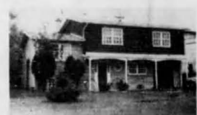
D.D.O.: $67,500 [36] 8 rooms, 4 bedrooms, nice family home on quiet street, westpart area. George Willie, F.R.I. 694-7540, 684-5040
