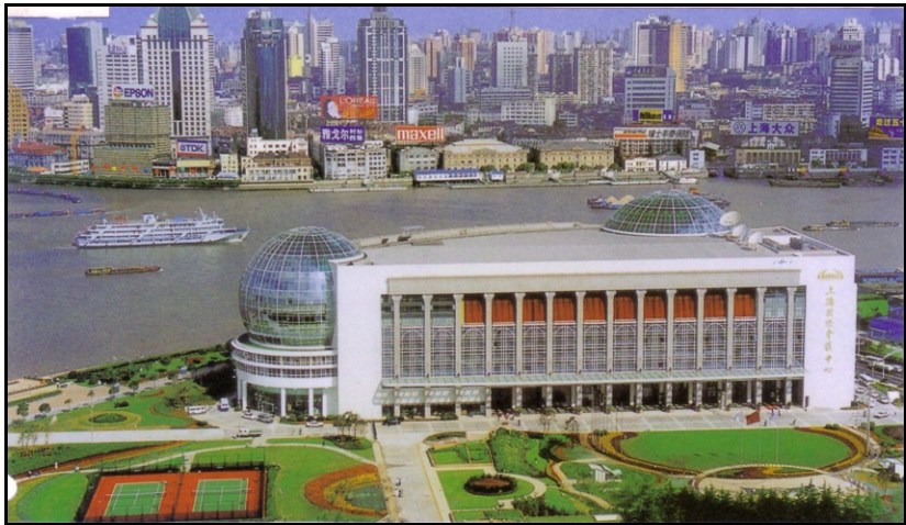
Figure 14.64: A shopping centre in Pudong.
