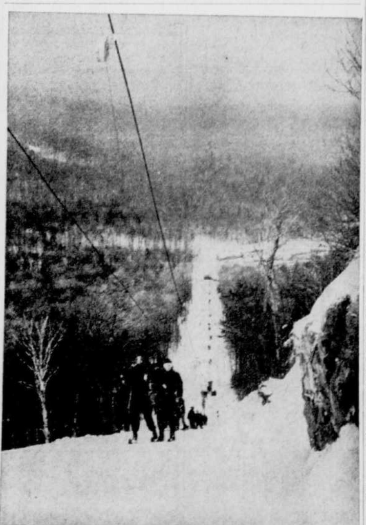
NEW SKI LIFT AT ORFORD —The new combination T-bar and chair lift at the Mount Orford Ski Centre went into operation last weekend. The first of its type on the continent. The lift is capable of transporting 800 skiers an hour to the summit of Orford's sister peak, Mt. Geroux "Little Black Mountain", 1970 feet above sea level. (Record Photo by Charles Catchpaugh)
