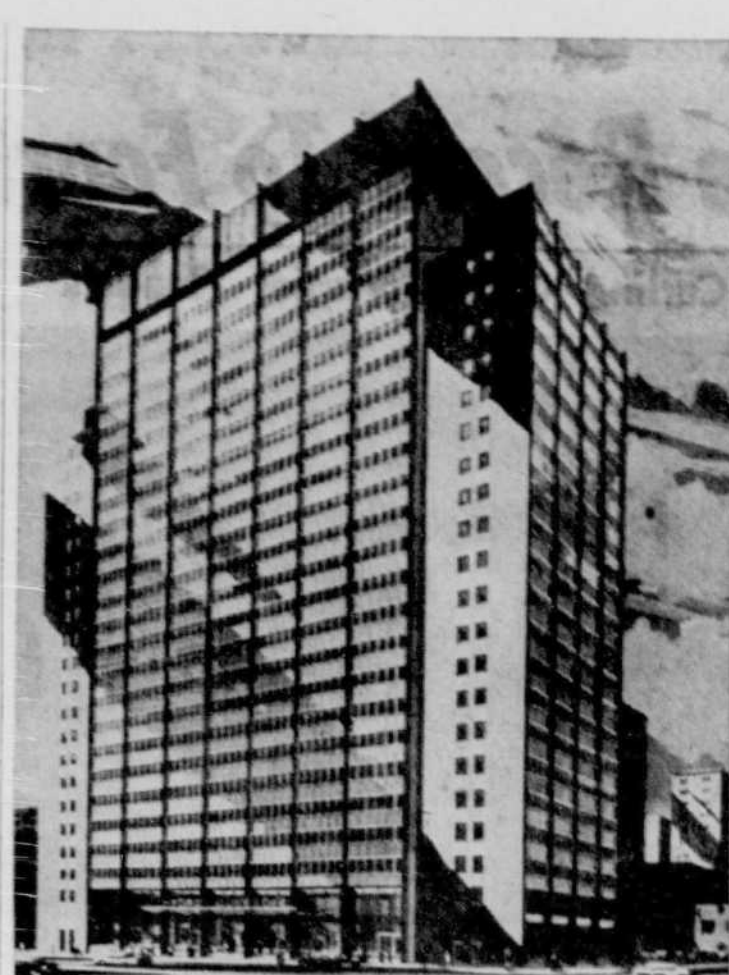
NEW QUEBEC HYDRO BUILDING — Pictured above is the proposed new Quebec Hydro-Electric Commission building to be erected on Dorchester boulevard, between St. Urban and Clark streets in Montreal. The building will feature an underground substation, purportedly the largest in America and will have five subterranean floors of parking space, capable of accommodating 250 vehicles. Building and substation are expected to be ready by the end of 1960.
