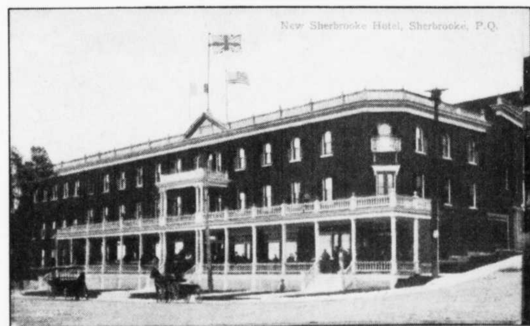
When the New Sherbrooke Hotel, Sherbrooke landmark, looked like this.
