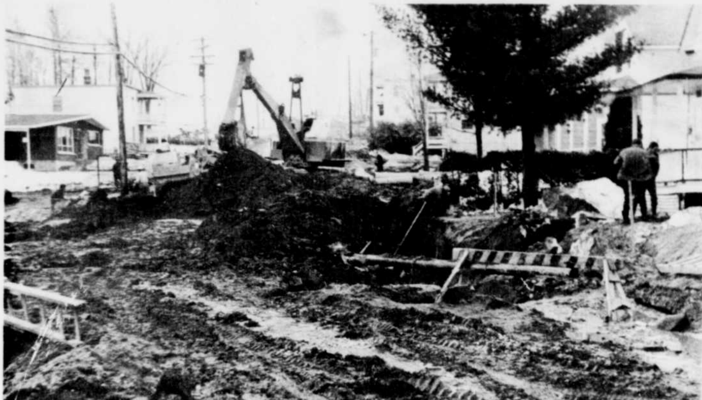
ROAD CLOSED — Belvedere Street south near the Sherbrooke city limits was closed to traffic yesterday as men worked to install new sewer pipes. As spring and summer begin to merge, roadwork starts again in the city. The road is supposed to be open to traffic today. (Record Photo: Crosbie Cotton)
